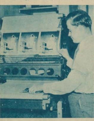
12 After the prints are developed, and "fixed" in hypo, Dick Schroeder dries them on cloth by heat & air in this machine
